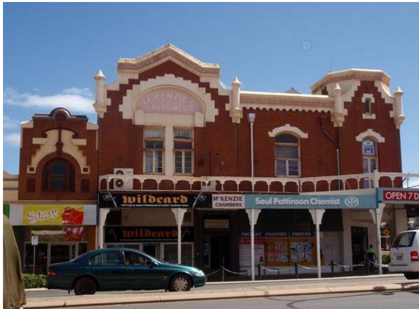
Hannan Street frontage of McKenzie's Buildings at Kalgoorlie, designed by Hawkins and Sprigg in 1904 (Penny O'Connor 2009, HCWA 01295).
