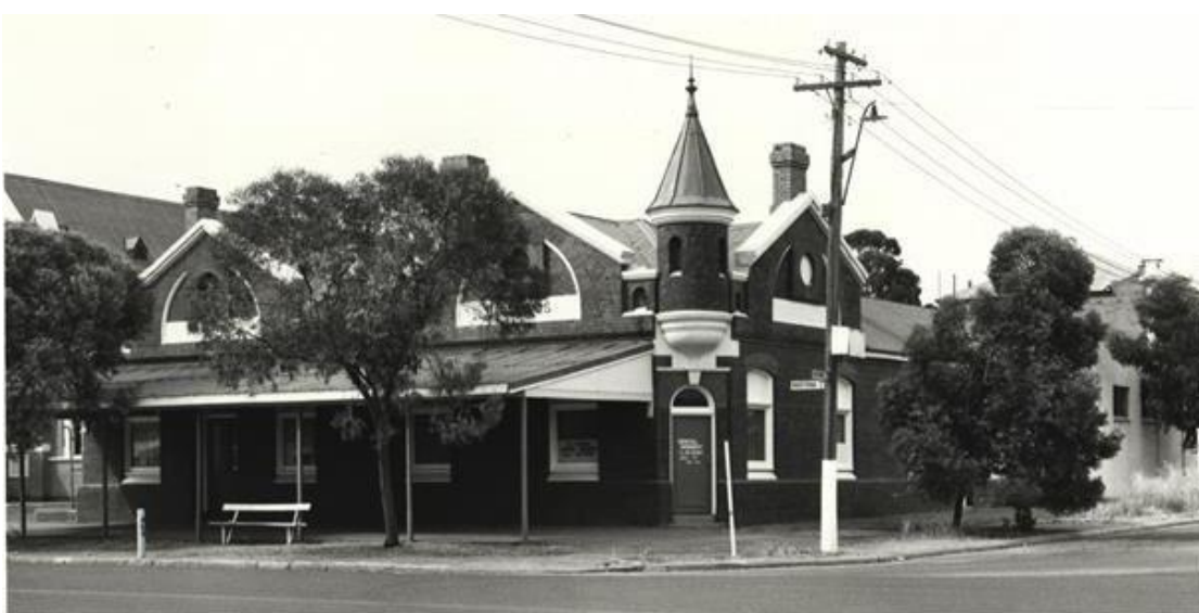
Maritana Buildings at 40 Brookman Street in Kalgoorlie, were designed by Hawkins and Sprigg in 1902 (F.A. Sharr 1982, HCWA 01319).
